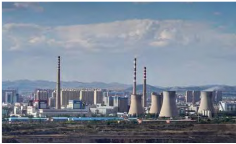
Incineration power generation
