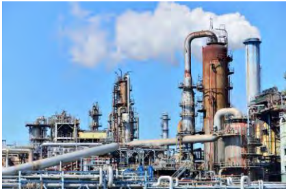
Petroleum and Petrochemicals
