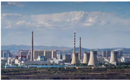
Incineration power generation
