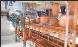
Ammonia leakage inspection
