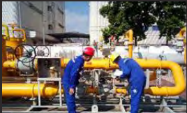
Natural gas inspection
