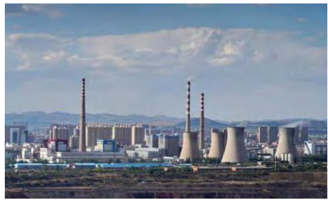
Incineration power generation
