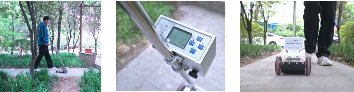
Leak detection of gas buried pipelines used for auxiliary roads, courtyards, and roads inaccessible to vehicles.
