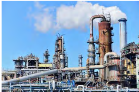
Petroleum and Petrochemicals
